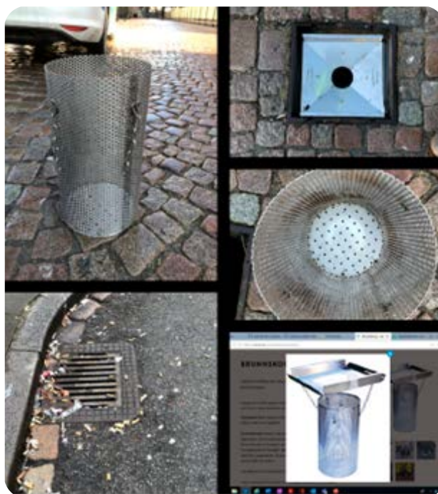
Figure 9: Basket devices from the company Reniva are placed under the lids of stormwater wells to collect cigarette butts
